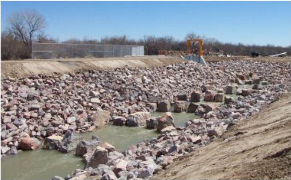
Figure 5-Public Service Company of New Mexico Diversion Dam Rock Fish Passage on the San Juan River, New Mexico
